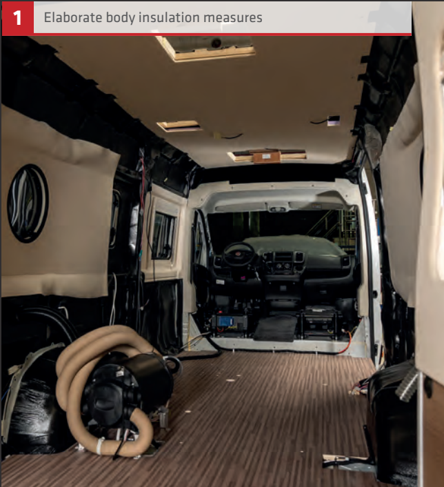
2 Side walls and main body frame members lined to prevent cold bridges
